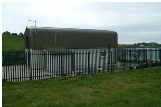
Dernakesh water treatment plant
